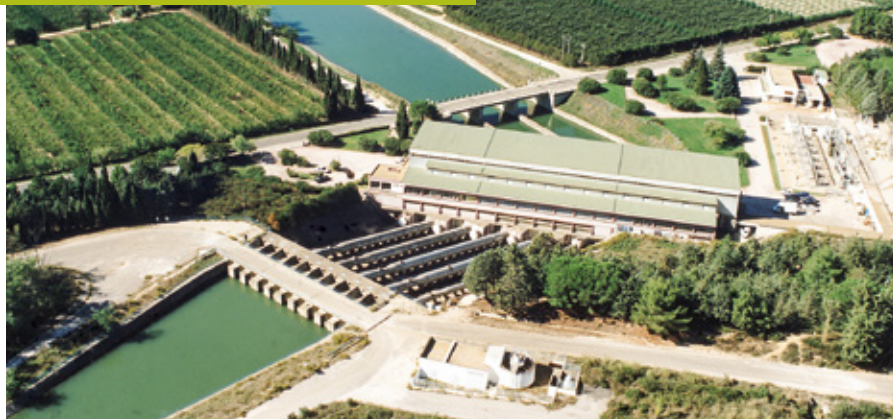
Station de pompage Aristide Dumont
